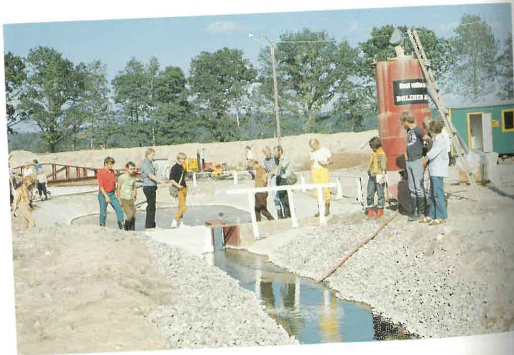
Figure 6. Lake Trummen. Plant for treatment (phosphate precipitation through addition of aluminium sulphate) of run-off water from the settling ponds. Photo: Sven Björk 1970.
