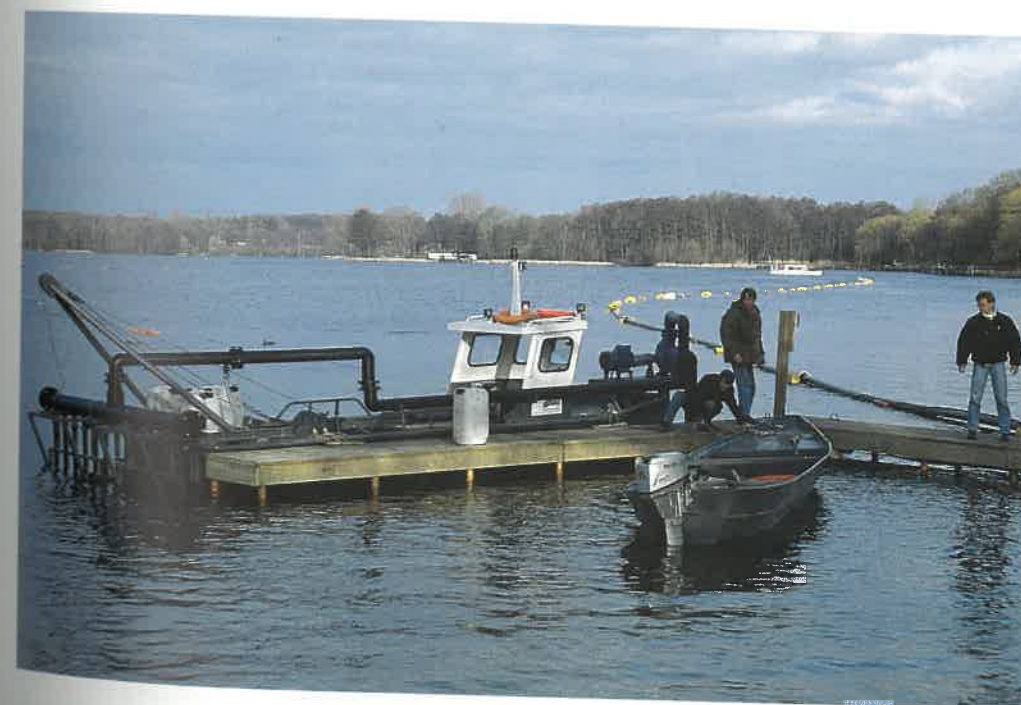
Figure 2. A floating tube is used for the distribution of iron oxide-hydroxide and iron chloride which are applied by a harrow from the boat to the lake.
